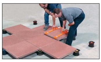
9- Run two or three lines of pavers down the center of the deck running in the opposite direction of the previously set pavers as noted in Caption 8.
