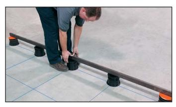
3- Make sure tops of the Line Course pedestals touch the bottom of the straight edge, this will help ensure proper pedestal height and levelness.
