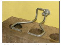
Apply adequate pressure to drive anchor until seated with head oriented as shown. **CAUTION:** Overdriving of anchor may cause thread stripout and inadequate pullout.
