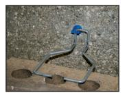
Drive Tapcon Brick Tie Anchor until fully seated and head slot is aligned horizontally as shown.
