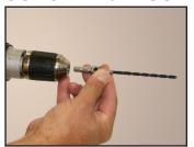
Place carbide bit into Condrive 500 drill adapter and tighten set screw. Place drill adapter into chuck of a hammer drill. Drill hole a min. of 1/4" deeper than thread length of anchor.
