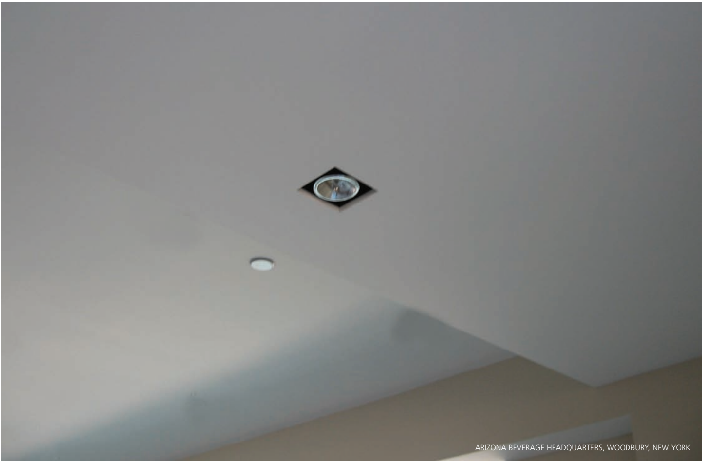
ARIZONA BEVERAGE HEADQUARTERS, WOODBURY, NEW YORK
