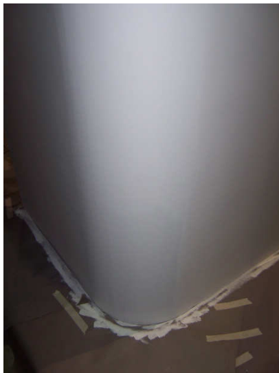
Finish & Prime like drywall
