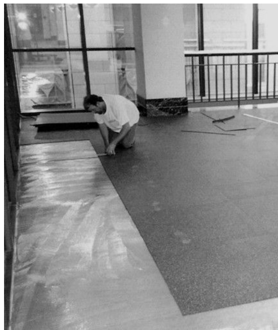
Square Cut Glue Down Installation
