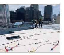
reduces the chances of board fracture that often occurs at the base of fastener stress plates. This is especially true with a fully adhered torch down application such as this."
