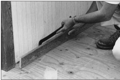
Carefully remove all existing wall base, trim, and transition moldings using a pry bar.
