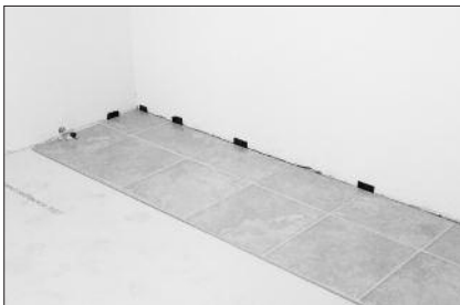
After careful planning and layout, begin by dry-laying the first row. Always work from left to right in the installation area and against the tongue side of the panel with the groove edge facing the wall. Whenever possible, avoid working directly on top of the panels because damage may occur. Maintain an expansion gap of 5/16" by using spacing wedges in the corners and where panels join together. If the starting wall is irregular, the first row must be scribed, cut, and fit to the contour of the wall.
