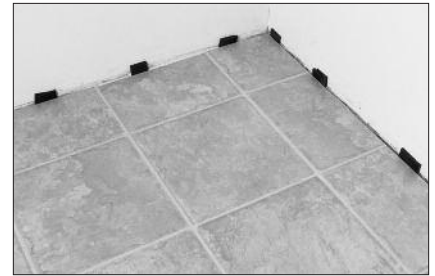
As with all tile formats, the best appearance is achieved by "balancing" the tiles at both the end and side walls. This can be accomplished by finding the centerline of the work area and adjusting the panels to provide equal size tiles at all walls.
