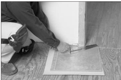
NatureForm Tiles must be installed over a Mannington Laminate underlayment such as AquaBarrier™ II, ComfortBarrier™ or Mannington® Hush. If you elect to use the Hush underlayment, be certain to take into account the additional thickness when undercutting door casings. Use a scrap piece of the new NatureForm Tile flooring as a guide. Be certain to allow enough room under
