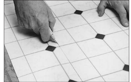
Follow the pencil marks on the surface of the resilient with a knife or scissors. Use caution so you don't damage the underfloor you're working over. A hookblade utility knife may make this easier.
