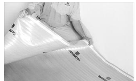
Install one sheet of AquaBarrier™ II underlayment net along the starting wall. Unroll only one sheet at a time during plank installation to prevent damaging the underlayment. If any part of the AquaBarrier II underlayment is punctured or damaged during installation, seal the area with duct tape.
