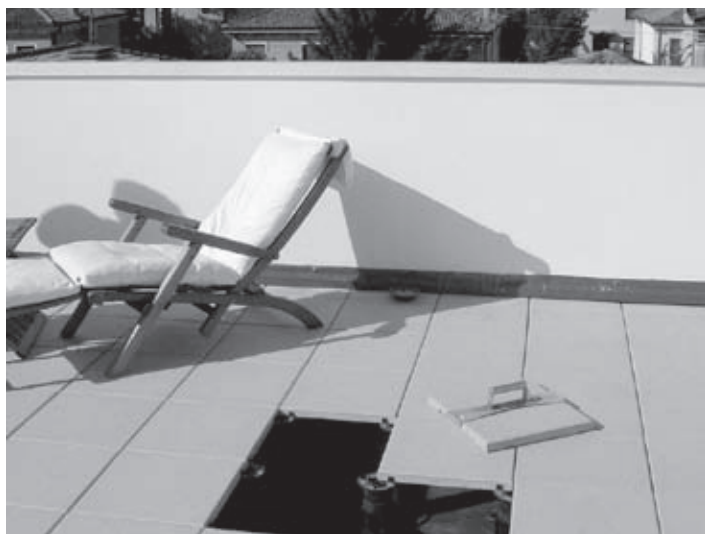
Private terrace - concrete tiles on Eterno pedestals
