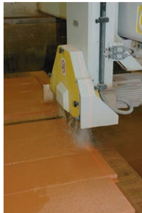
Multi-axis Saw Cutting Tiles
