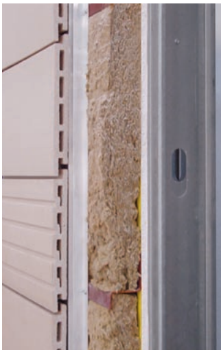
Typical Panel Section
