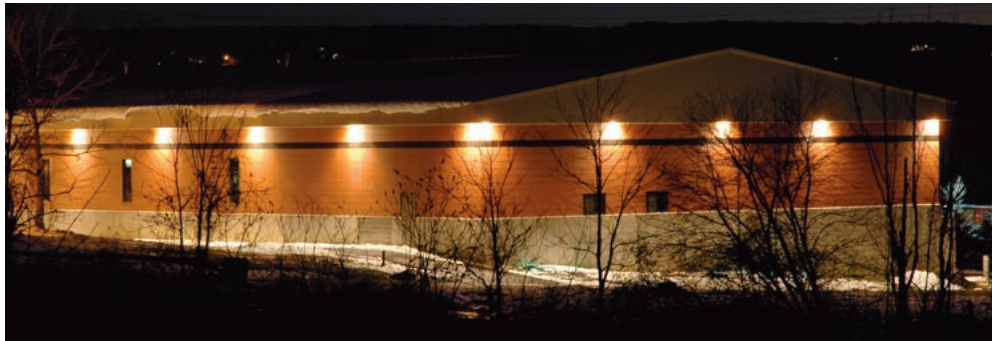
TerraClad Production Facility
