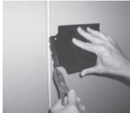
Tab Removal – Right Hand Application
