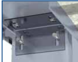
Attach DriftClip DSLD to stud with provided #8 screws through each Step Bushing.
