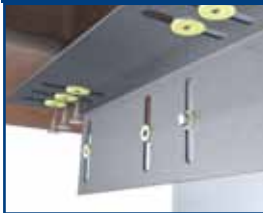
Attach DriftClip DSLS to structure with specified fasteners through step bushings.
