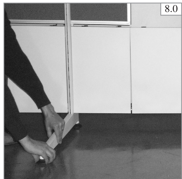
FreeWalls nivellieren. Level out FreeWalls. Niveler l'ensemble.
