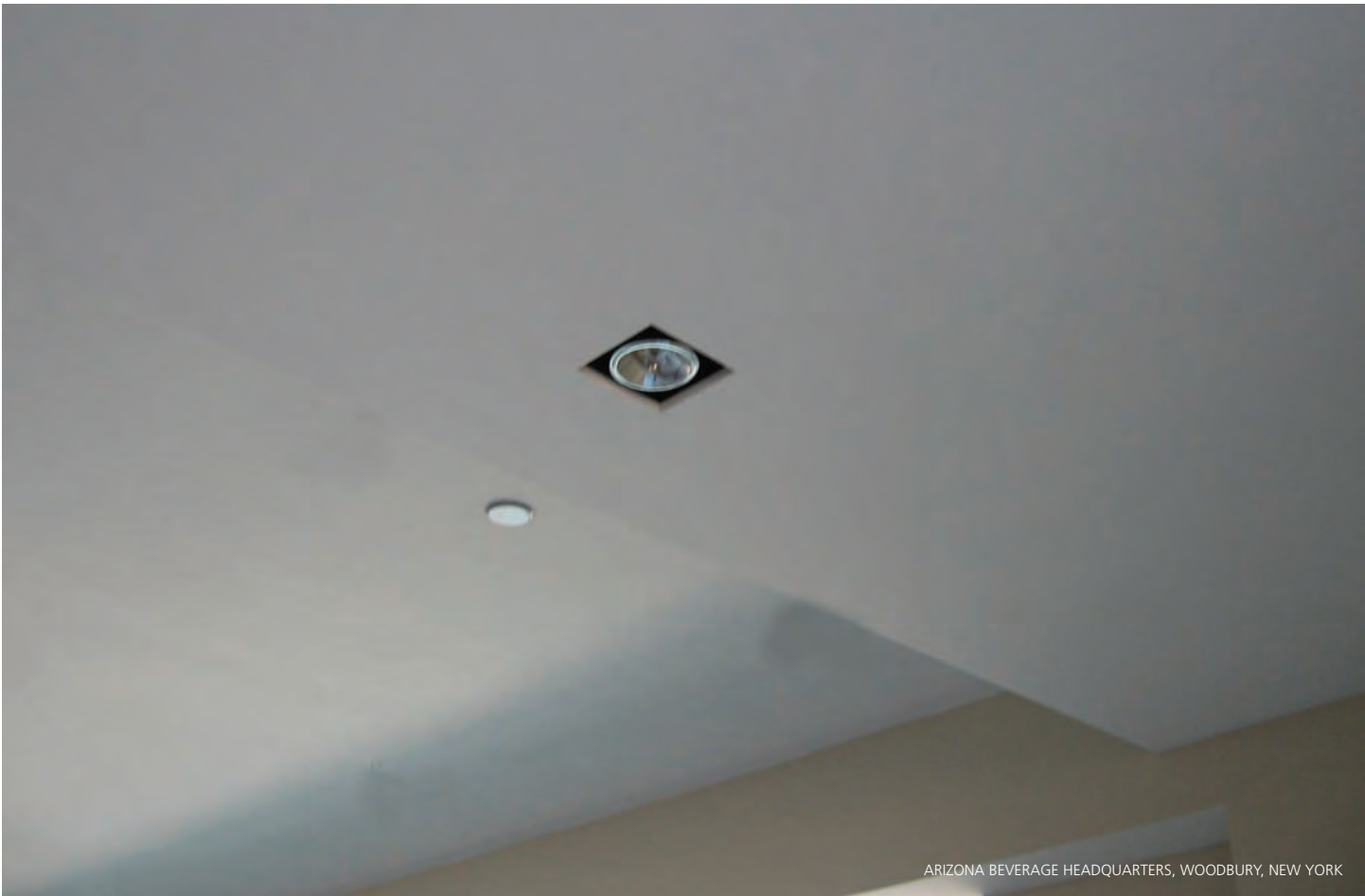
ARIZONA BEVERAGE HEADQUARTERS, WOODBURY, NEW YORK
