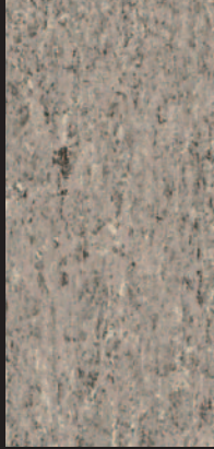
LP164 falling rock
