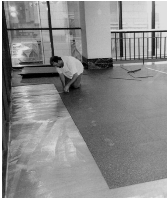
Square Cut Glue Down Installation
