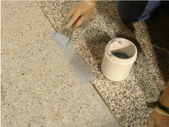
Apply FUSION™ to joints
