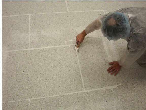
Remove excess FUSION™
