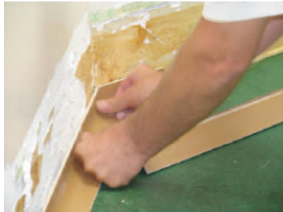
Secure base into position with adhesive
