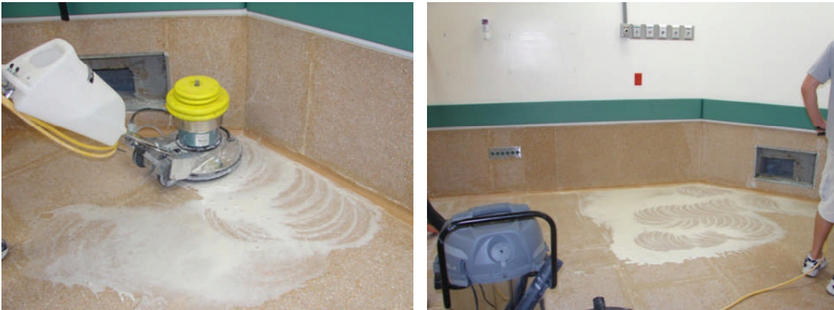
Wet-polishing procedure to remove residue and eliminate lippage.
