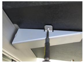
Tighten the cap screws that attach the power island to the main beam.
