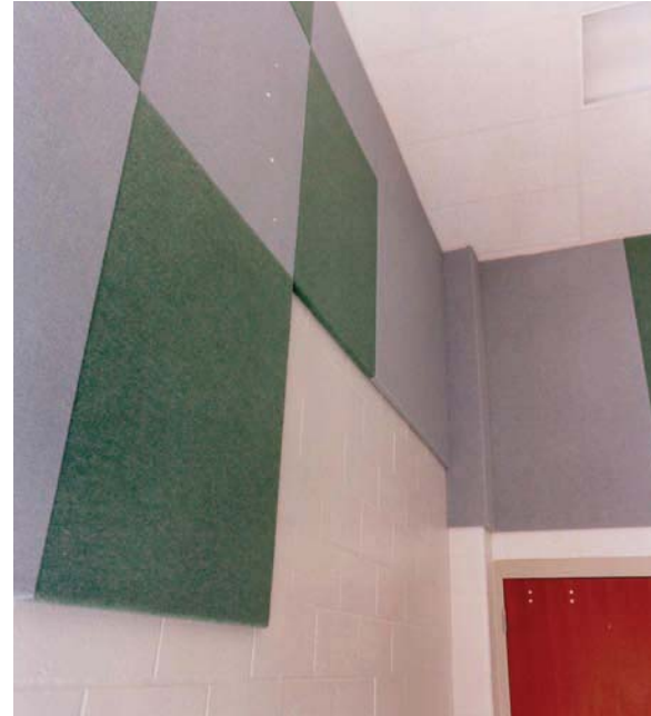
Fabri-Tough Wall Panels are mounted using the internal spline system.
