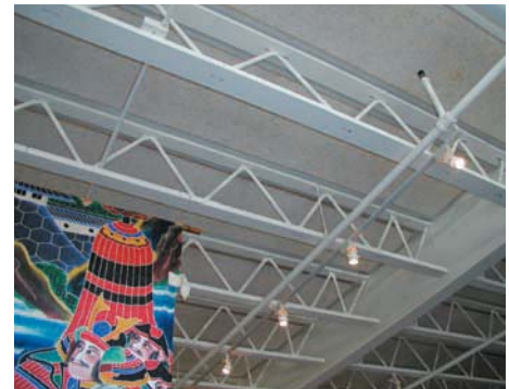
Beacon Building (Culver City, CA) ▶ Direct-Attached Ceiling Panels
