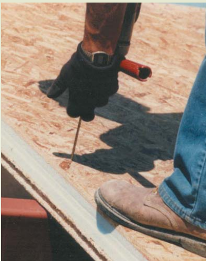
Tectum E installed over steel. ▲
