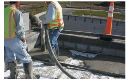
▲ Installation of lightweight insulating concrete over a Tectum I roof deck.
