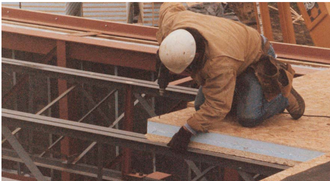
Tectum III Installation
