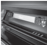
Power Distribution Unit (Rigid Wireway)
