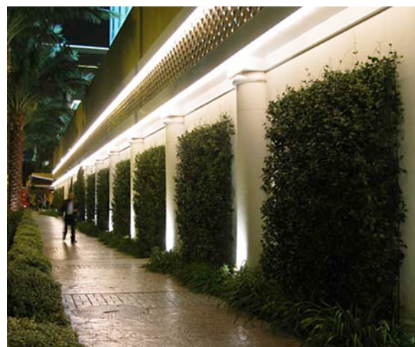
Multiple, three-dimensional panels with easy maintenance access help to reduce reflected light and heat gain in an arid environment, Las Vegas, NV
