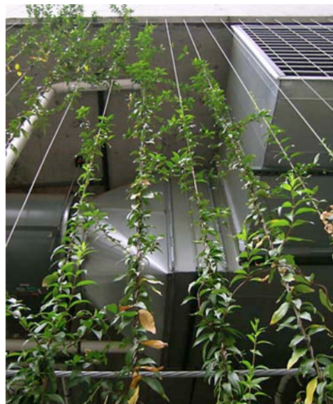
Two-dimensional stainless steel cable system with long vertical spans, Dallas, TX
