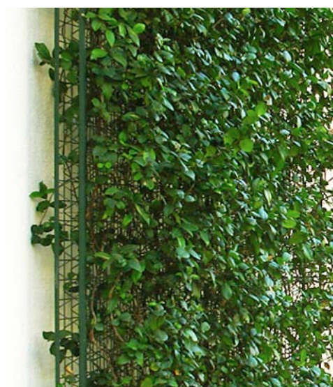
Wall mounted, modular, three-dimensional panel with mature growth
