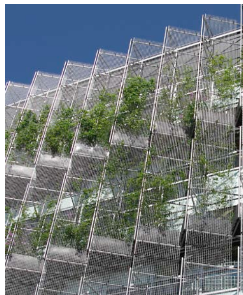
Modular, three-dimensional green facade system adapted to a tubular steel frame with integrated planters and irrigation, Vancouver, B.C.
