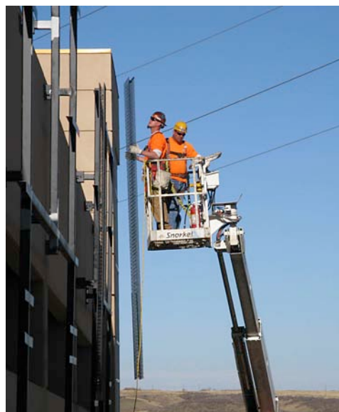
Rigid, lightweight, three-dimensional panels being installed on a multilevel building, Golden, CO
