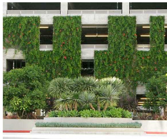
Surface-mounted green facade with plants trimmed to panel edges, Playa Vista, CA
