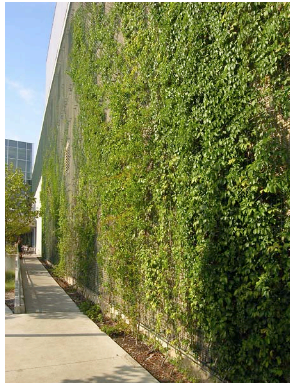
A wall mounted, modular, three-dimensional, green facade system, Chicago, IL
