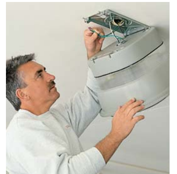
Hanging from the tab, luminaire is wired...
