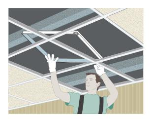
Next, drop the SkyTile into the Elevator.
