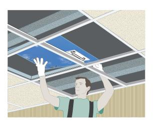
Then set the EcoSlim light box on top the Elevator/SkyTile sandwich..
