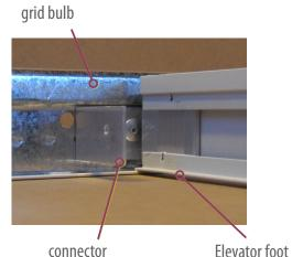
Bend connector as needed to fit the angle between grid and perimeter.
