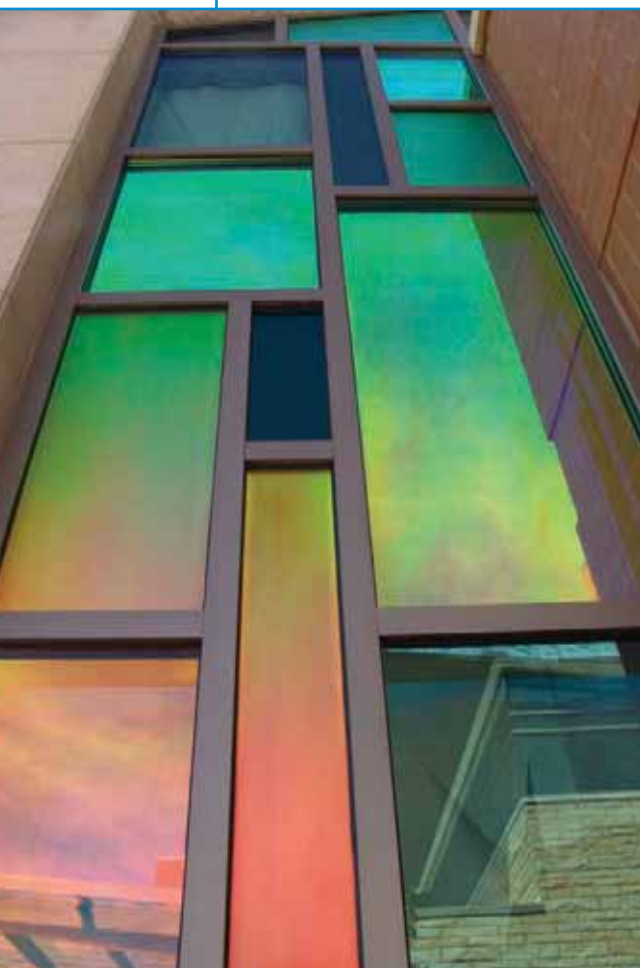
John Blazy's decorative glass can be seen in a range of applications, including the TriPoint Medical Center in Concord, Ohio, which features Dichrolam red insulating glass units.
