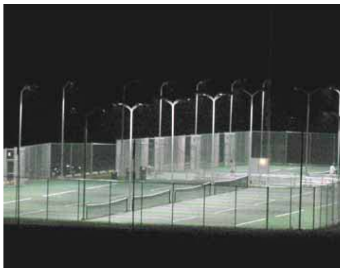
Full cutoff lighting produces more useable illumination.
