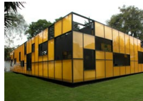
PANELITETM IGU/TO-4 • Falcón Headquarters, Mexico City, Mexico • Design: Rojkind Arquitectos Photography: Panelite
