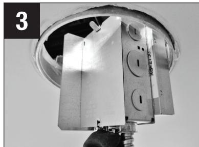
3. Insert LED driver box thru ceiling cut-out and rest driver-side up.
