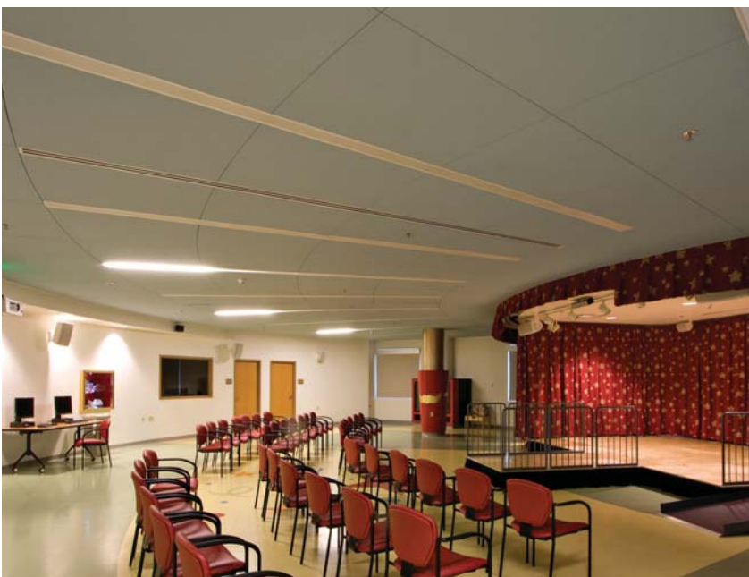
Custom colored radial ceiling panels suspended with Ceilencio.
