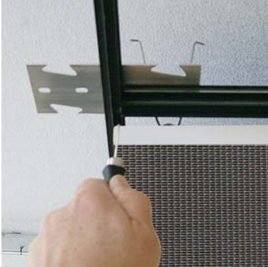
Pull down gently keeping tool engaged behind panel until panel edge can be held with free hand.
