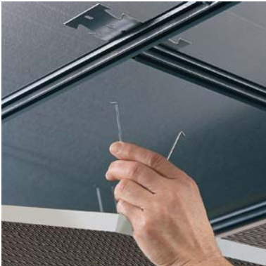
Disengage panel retainer springs from "butterflies".
