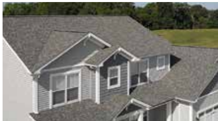
ROOFING AND VENTILATION
