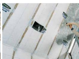
High performance loose-fill insulation designed for installation into framed construction cavities covered with non-woven OPTIMA® fabric or equivalent.
