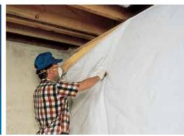
Half-wall or full-wall insulation available in two facings, white PSK and standard FSK. Designed for use in both residential and commercial applications where code or builder preference specifies an insulated basement area. Both facings are perforated. Intended for applications where insulation will be left exposed.
