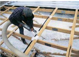
High performance fiber glass blowing insulation. Designed for installation in open or closed cavities. Lasts for the life of the building to reduce energy demand and costs. Applied using recommended pneumatic blowing machines.
