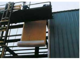
A flexible blanket of fiber glass insulation, furnished in rolls. It can be faced on one side with a suitable vapor retarder by independent metal building insulation laminators.
