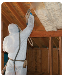
Spray Foam Insulation
