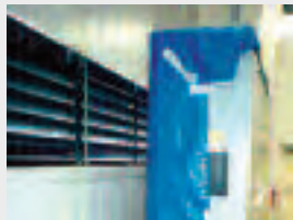
Rain coming through louvers can cause critical building equipment and systems to fail. Specify Storm Resistant Louvers.
