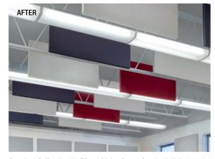
Soundsoak Baffles 2' x 4' in FR-701 fabrics; Custom Soundsoak Walls 3.5' x 3.5' with Mineral Fiber substrate and Square Edge in FR-701 Silver Papier fabric.
