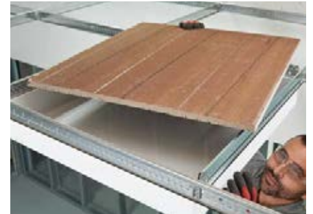
MetalWorks™ 3D ceiling panel with School Zone® Fine Fissured™ 1713 acoustic infill panel for Total Acoustics® performance
