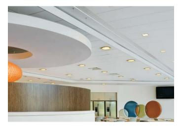
This pre-engineered vertical trim solution for 5/8" drywall eliminates vertical framing and provides architectural detail.
