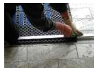
Overlap the mat well frame and cut with ruler and knife
