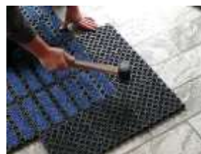
Assemble tiles with a hammer or rubber mallet(*)
