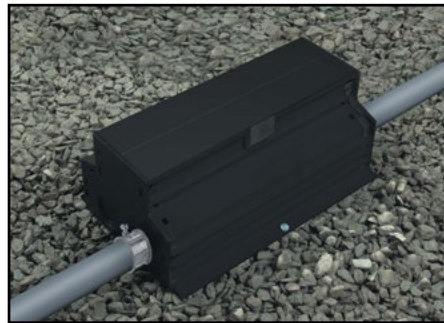
Install electrical components. Level and anchor blockout with retainers
