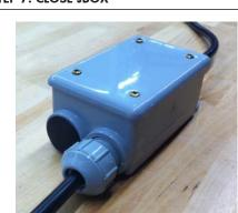
CLOSE THE JBOX USING THE GASKET AND COVER PLATE (4X SCREWS INCLUDED).
