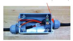
BE SURE TO LEAVE A MINIMUM 3" LENGTH OF CABLE AND WIRE LEADS INSIDE THE JBOX TO MAKE CONNECTIONS
