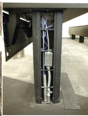
J Box can be mounted inside table base or the base can mount over some flush mounted floor boxes
