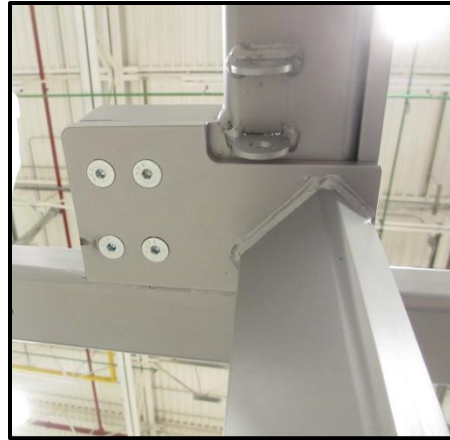
Note: Leg Attachment using provided fasteners
