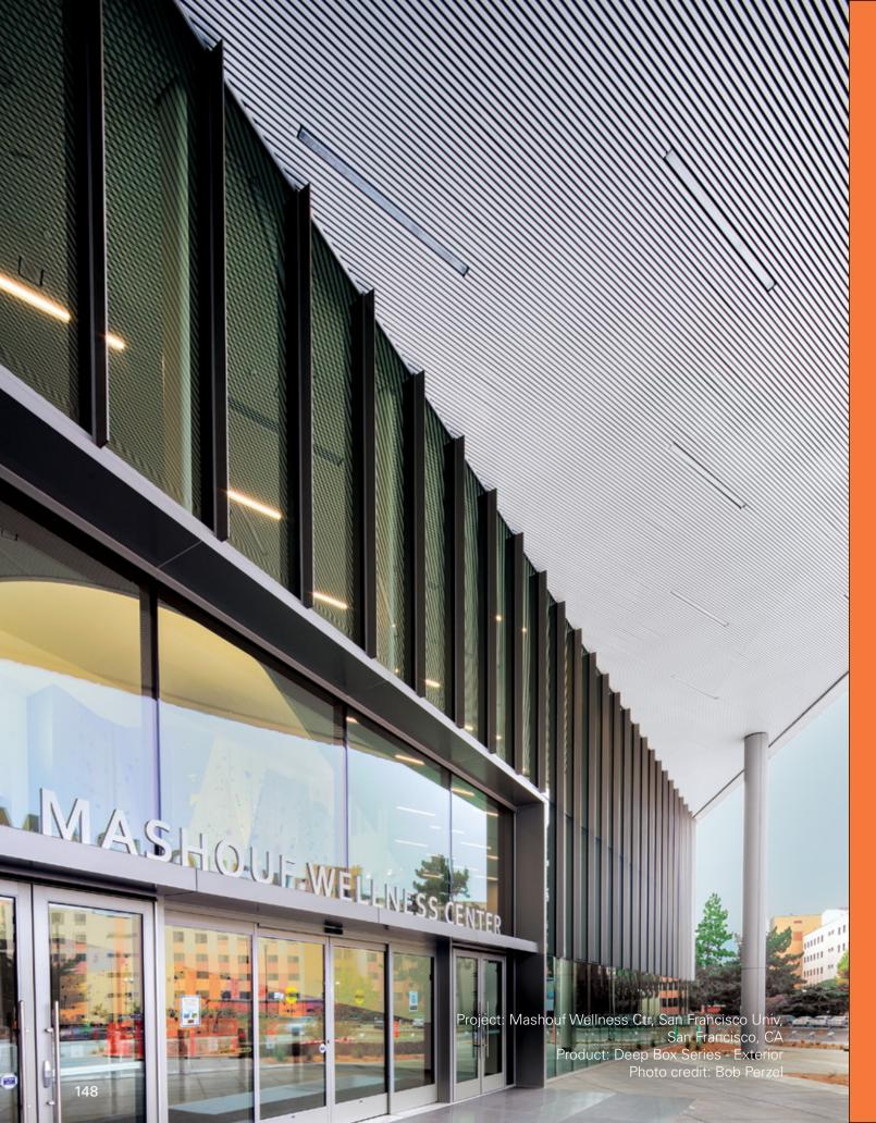
Exterior Soffit ceilings create a variety of distinct looks and are engineered to withstand harsh environments.
