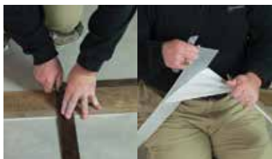
Cut flooring with coated release paper in place
