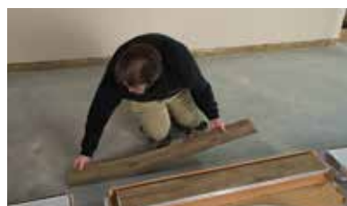
Install pieces by holding both ends
