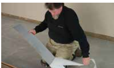
Stage products for design variety and begin by removing coated release paper
