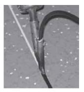
noraplan® floors do not need to be welded, with the exception of noraplan® acoustic, which does require welding due to its resilient structure.
