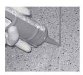
It is advisable to seal joints in case of moisture-sensitive subfloors, in rooms permanently undergoing intensive wet cleaning, or in areas with special hygienic requirements. For these special requirements, the sealing of all norament® and noraplan floorings is suitable, with the exception of norament® 992 and norament® 992 grano.
