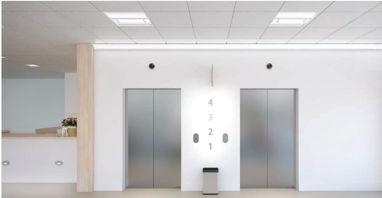
Flexible Ambient provides general ambient lighting with adjustable accents to highlight signage and add extra dimension in an elevator lobby.
