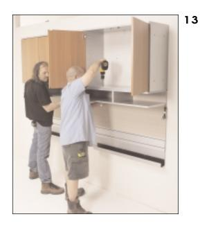
Position the lower storage unit with lights. Fasten with woodscrews through predrilled holes inside overhead. Install shelf pins into middle set of holes. Insert shelves.
