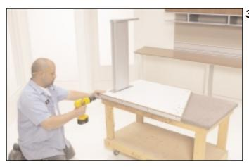
• Install pencil stop as previous (no rubber extrusion on this top).
