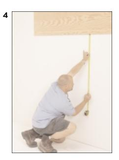
Measure down 27<sup>3</sup>/16" from the bottom of the plywood cleat. This point represents the bottom of the aluminum cleat.
