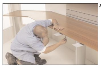
For optional fixed top, install flat brackets to main work surface. Note this top has two positions for installation. Choose bracket locations furthest away from the closet. 37 38
