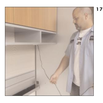
• Feed the lighting cable into the top slot at the closet back and out of the bottom slot.
