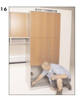
From the interior of the cabinet; level the closet, aligning the holes for attaching the overhead storage unit.
