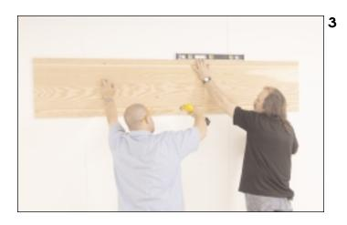
At the bottom of the plywood cleat, mark centre and position it at the centre point on the wall. Level and appropriately fasten the cleat to the wall.
