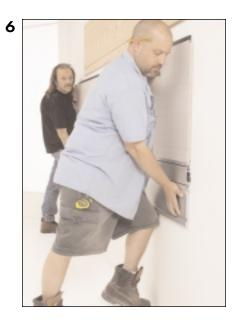
• Slide the tack panel assembly onto the aluminum cleat.
