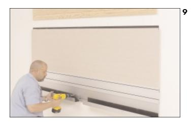
• Apply the wire management to the bottom of the panel with wood screws.
