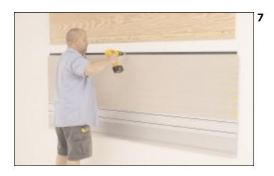
• With wood screws, fix the top of the assembly into the predrilled holes.
