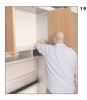
• Attach the overhead to the closet with hardware supplied.
