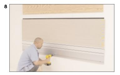
• With wood screws, fix the bottom of the assembly into the slot provided. DO NOT install wood screws in the centre 12" of this slot.
