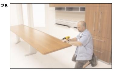
• Install aluminum pencil stop through predrilled holes with wood screws. Justify the stop flush against closet edge and 3/8" above work surface.
