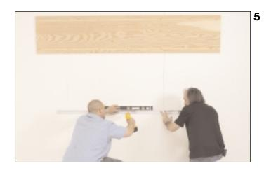
• Centre and level the aluminum cleat. Fasten appropriately.
