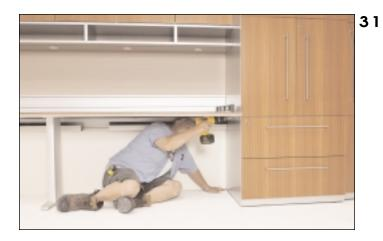
• Adjust level as required with bolts in slots and lock bracket in position with two woodscrews.
