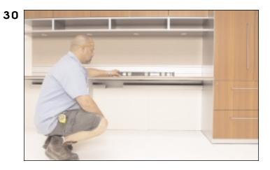
• Fix top to bracket with threaded bolts supplied.
