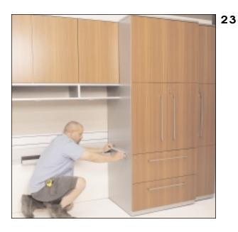
• Install top bracket to closet with 3 machine screws into 3 slots. Flat side of bracket to the top.
