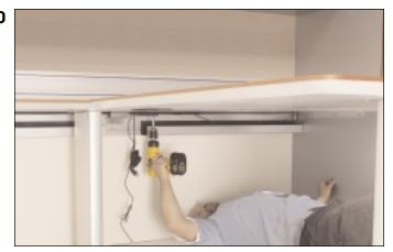
• Plug lighting cable into transformer assembly and mount the transformer to the underside of the top with woodscrews.
