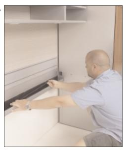
• Lay the lighting cable in the trough.
