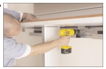
Apply top to wall bracket in the gap between the wire troughs. Additional bracket is required along wall past tack panel – install into metal stud.
