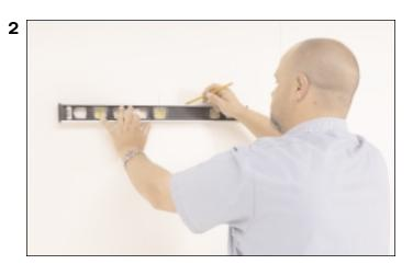
• From this point, mark a horizontal level line roughly in the centre of the wall.
