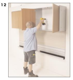
• Install woodscrews through the interior of the overhead, locking it to the plywood cleat.
