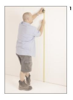
• From the highest point in the room, measure up from the floor surface 59<sup>7</sup>/8". This dimension will mark the bottom of the wood cleat.
