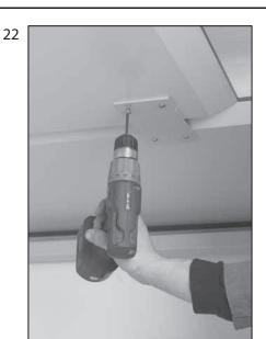
Place return top in position, align the threaded inserts with holes in the bracket and install 1" x 1/4 - 20 flat head hex socket bolt.
