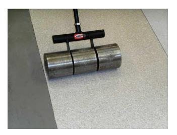
8. Cut the second sheet and position it so that the factory edge overlaps the previously installed edge by a minimum of 1/2".
