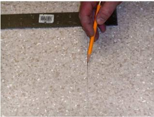
9.B. Using a recess scriber, cut windows along the edge of the seam. At a minimum, one window should be made at each end of the sheet. After cutting the window, establish cross reference points on the top of both pieces.
