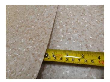
9.A. Using a pencil and small square, establish reference points onto the top of both sheets. One mark should be placed perpendicular to the seam and another should follow the edge of the overlapping sheet.
