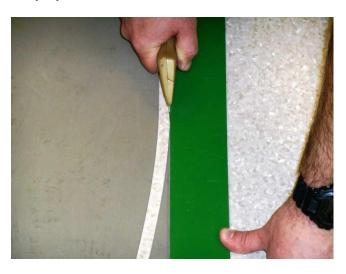
2. Move the sheet into position and mark a reference line onto the substrate following the
