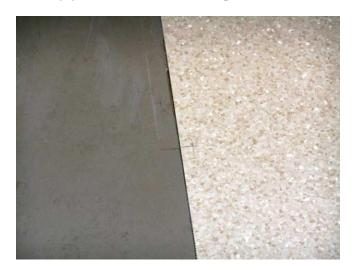
7. After laying the sheet into the adhesive, roll the floor in both directions using a 100 lbs., three-section roller.
