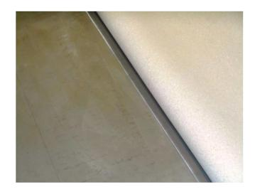
5. Using the correct trowel, apply the Tarkett adhesive onto the substrate. Follow the previously established reference lines when troweling adhesive.
