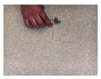
11. Place a piece of scrap material under the second sheet when cutting the seam. Utilize a utility knife with a sharp blade to cut along the scribe mark.
