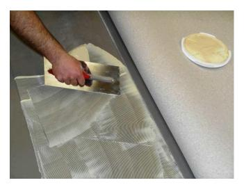
6. After the adhesive is allowed the appropriate open time, lay the sheet into the adhesive. Use the previously established reference marks to help position the sheet during installation.
